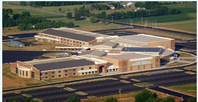
▲ **SOUTH WARREN MIDDLE & HIGH SCHOOL** (2010) THE LARGEST SINGLE STRUCTURE INSULATED CONCRETE FORMS BUILDING IN NORTH AMERICA & THE FIRST EDUCATIONAL PROJECT TO UTILIZE INSULATED CONCRETE FORMS CONSTRUCTION FOR BOTH INTERIOR & EXTERIOR BEARING WALLS.
