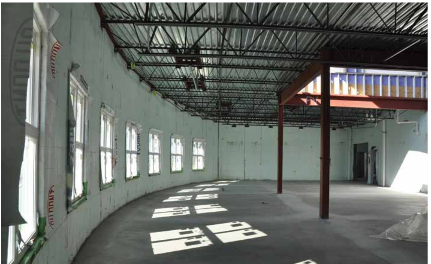
NUDURA Radius Forms are custom cut at Nudura's plant facility to meet the design specifications, then preassembled for easier and faster installation.
